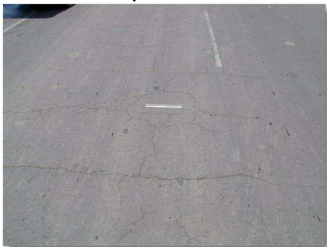
Figura 6: Fisura Transversal
