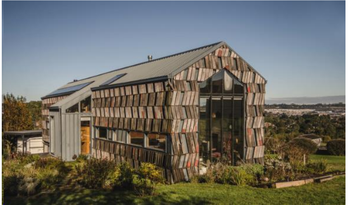
Figura 5 Casa larga María Laura Cristi +Tramarquitectura (Tomado de Arch daily, https://www.archdaily.co/co/924176/casa-larga-maria-laura-cristi-plus-tramarquitectura )
